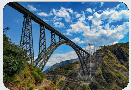
Chenab Railway Bridge, J&K (2024), world's highest single-arch railway bridge
