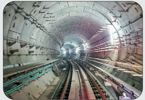
East-West Metro, Kolkata (2024): Consists of India's first underwater Metro tunnels, India's deepest metro station and country's deepest metro ventilation-cum-evacuation shaft
