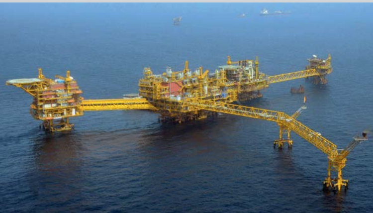
L&T's mega projects: The Mumbai High North Process Gas Compressor Modules (hydrocarbon) project.
