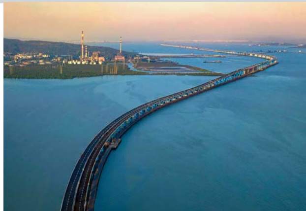
Mumbai Trans Harbour Link, dubbed India's longest sea bridge.
